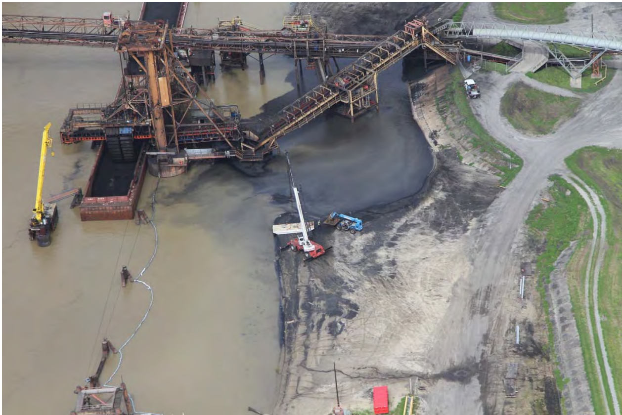
United Bulk Terminals Davant facility
